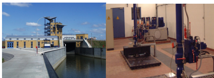
SONOCONTROL for position control at locks of a waterway in Middle Germany
